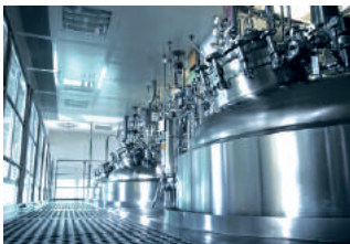
Tank and silo weighing
